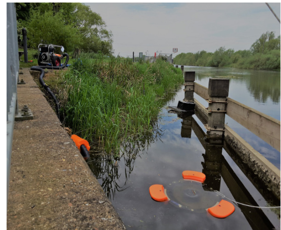
Above: Skimmer connected to VikoPump
